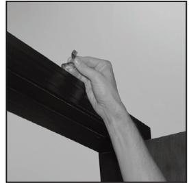
2. Position the bottom edge of the Plastic Bar(5) so it is resting securely on the hinge side of the door on top of the door frame/molding and on top of the Safety Wedge(19).
